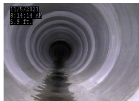
WASM 3 - cement-mortar lined steel pipe
