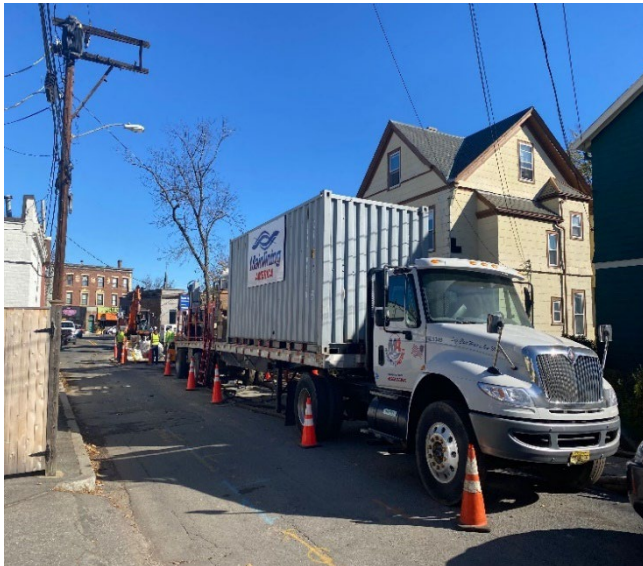
Cement Lining Equipment at Pipeline Access Pits
