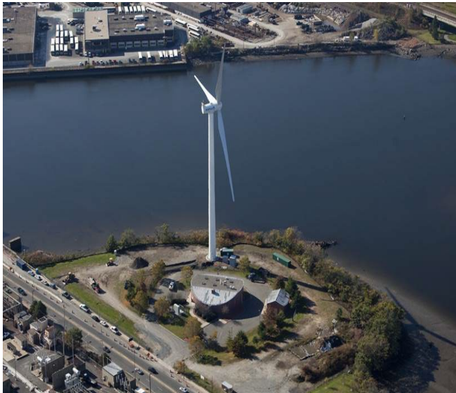
Figure 3: 1500 kW Wind Turbine at DeLauri Pump Station
