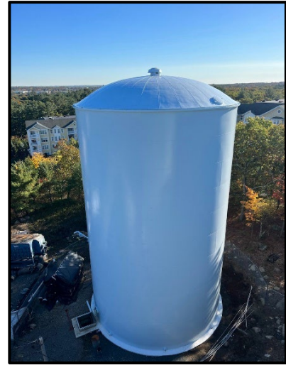
Rehabilitated Water Storage Tank
