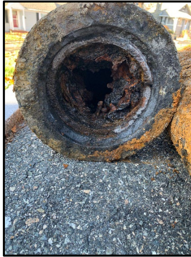
Cleaning and Lining Old Cast Iron Water Main
