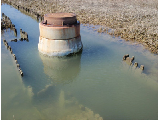
Sewer Manhole in Marsh: Raised and Sealed
