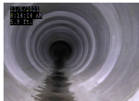
WASM 3 - cement-mortar lined steel pipe
