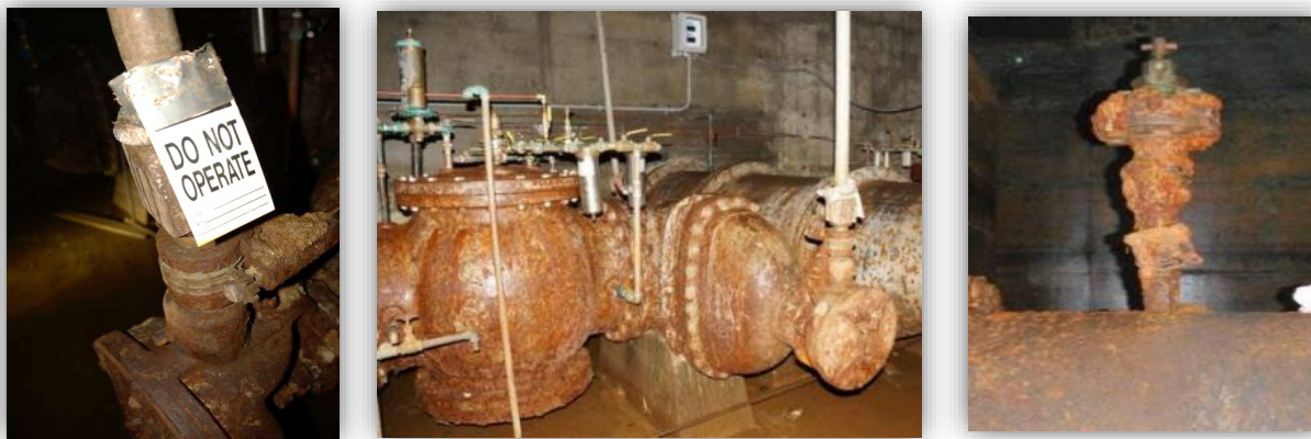
Figure 1 – Condition of Some Existing Tunnel System Valves
