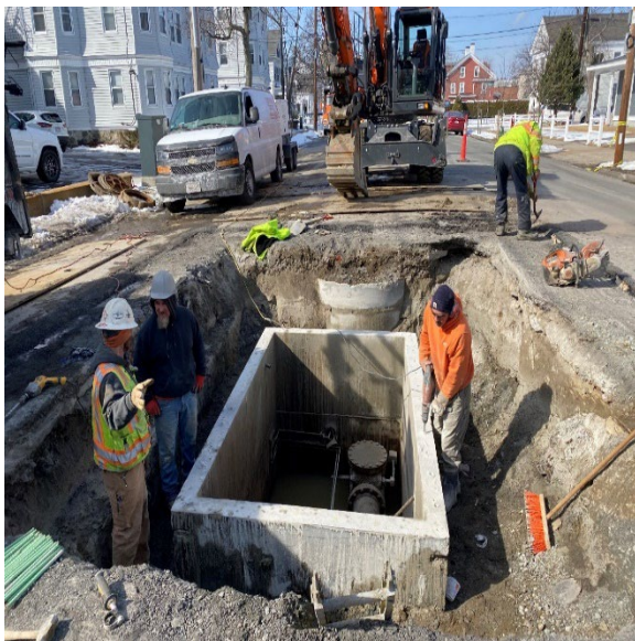
Cutting Concrete Walls at Meter 171
