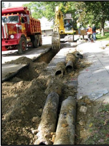
Water Main Replacement Construction
