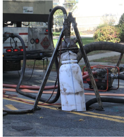
CIPP Liner Installation
