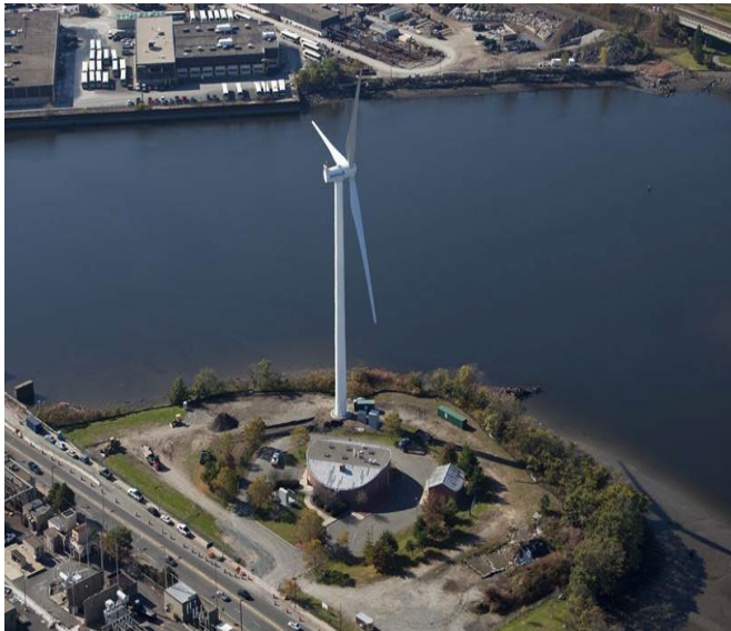
Figure 3: 1500 kW Wind Turbine at DeLauri Pump Station
