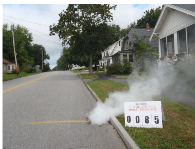
Inflow Source Identified by Smoke Testing
