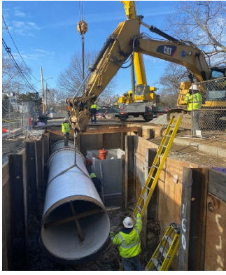
WASM 3 – pipe replacement
