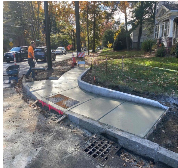
ADA Compliant Ramps at Pleasant Street
