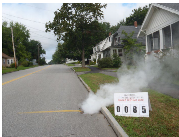
Inflow Source Identified by Smoke Testing
