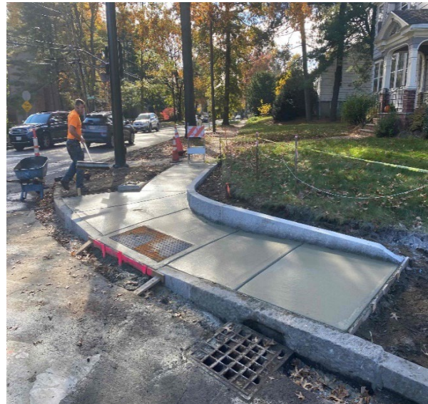
ADA Compliant Ramps at Pleasant Street
