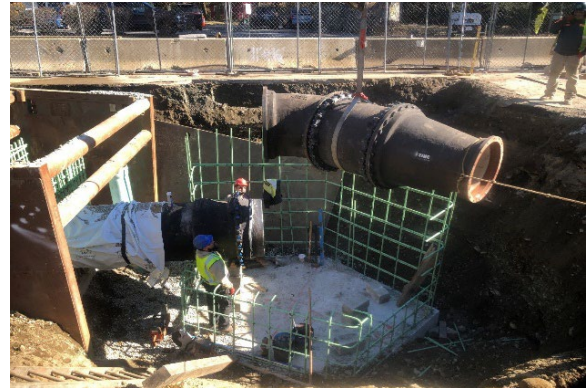
36” pipe & thrust block @ Lexington St & Totten Pond Rd
